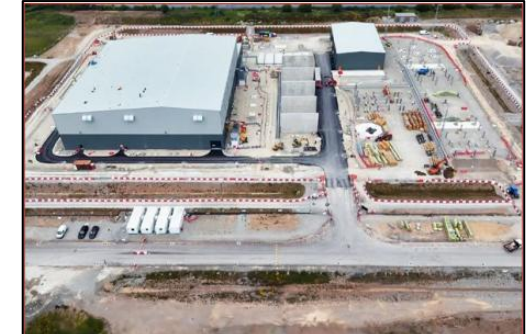
Interconnector Cable between Ireland and France
